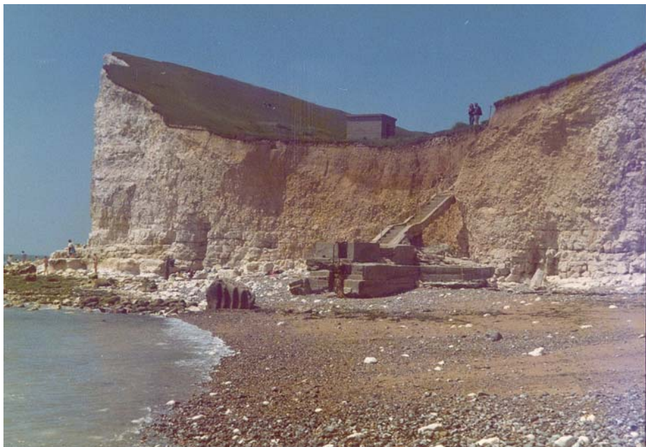
Figure 1: Old stairs at Hope Gap in 1979 (Lewes District Council)
