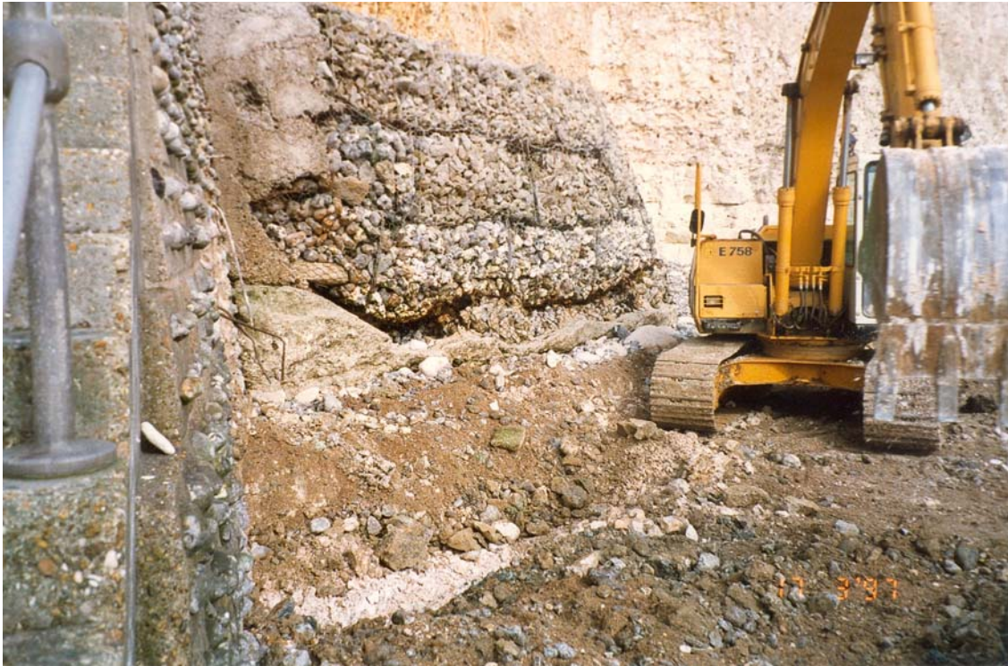
Figure 4: Excavator used in 1997 for the repair of the gabions to the east of the steps (Lewes District Council).
