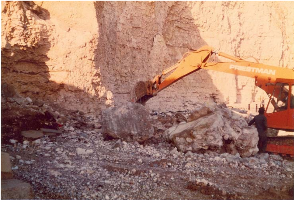
Figure 2: Image of the excavator used in 1979 demolishing the old stairs (Lewes District Council)
