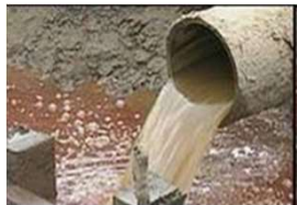
Sewerage collection without treatment
