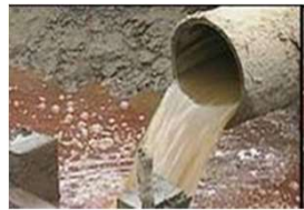
Sewerage collection without treatment
