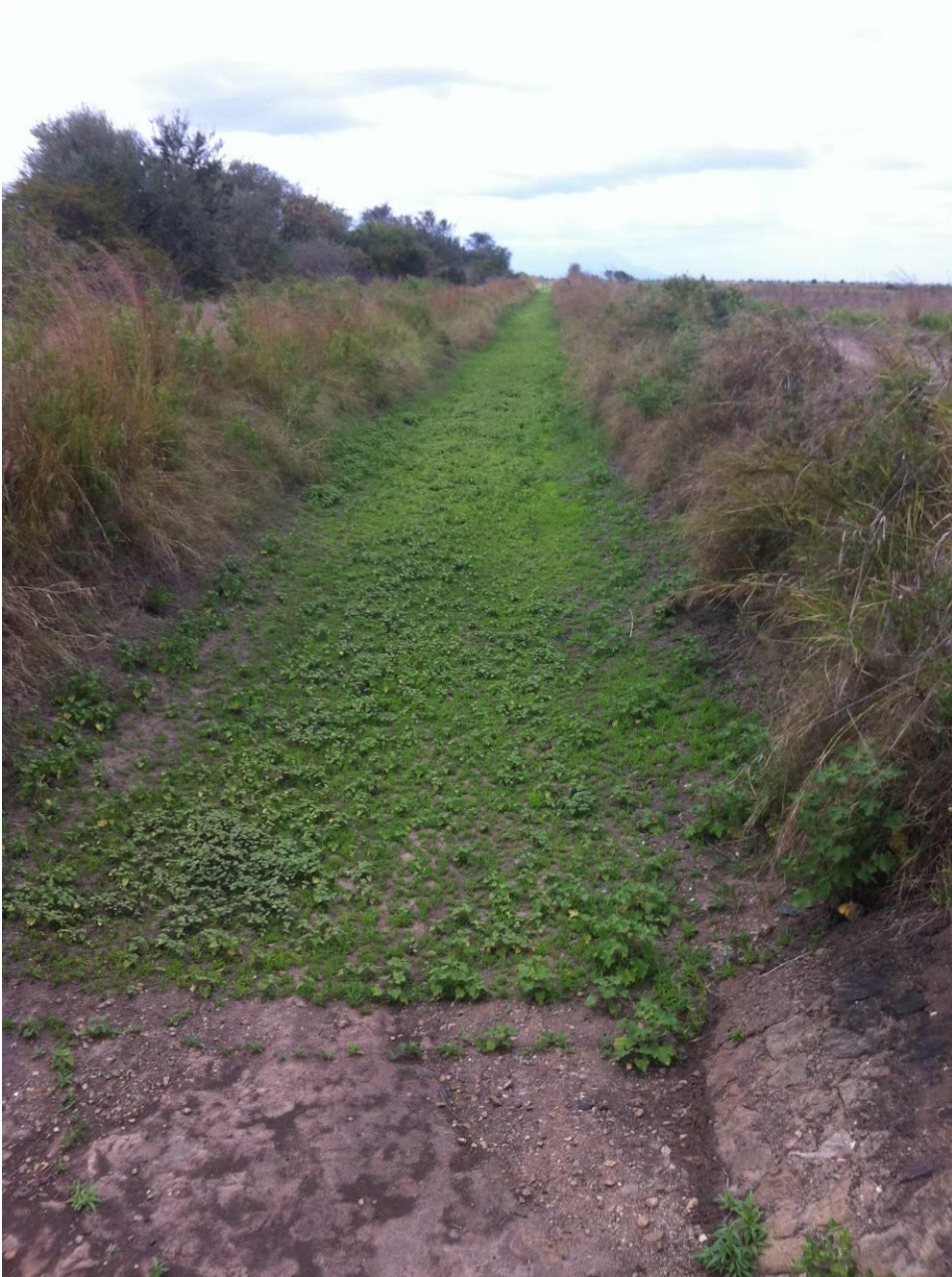
Main irrigation canal
