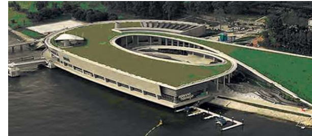
Wastewater recycling centre
