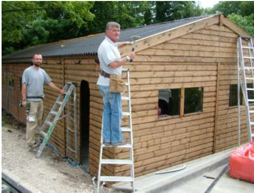
Builders constructing the workshop extension, which houses a honey bee extraction facility and a cold store
