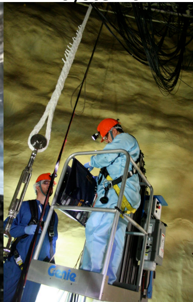
Installation of in-situ calibration systems
