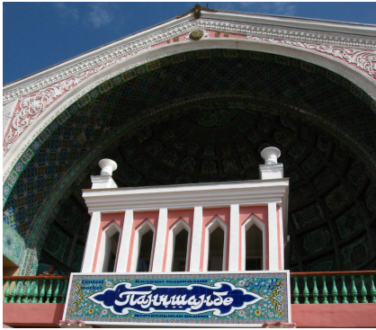
The facade of the Panshanbe market in Khujand
