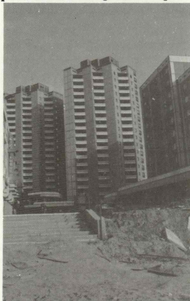
Tower blocks nearing completion, Marzahn, Berlin, GDR, 1989.
