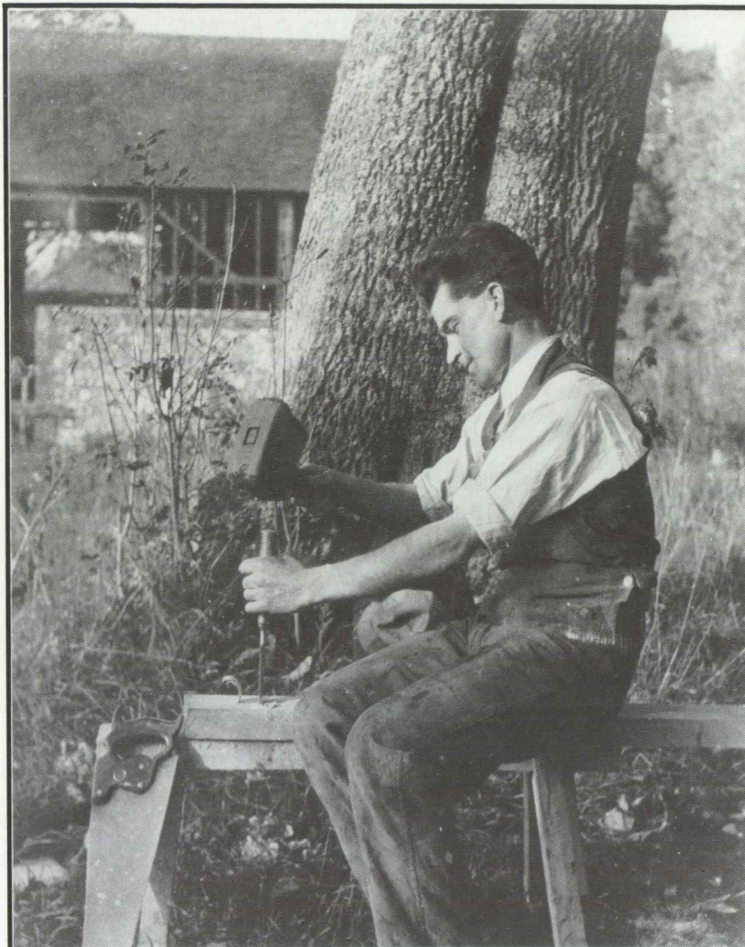
Owen Williams working outside Tenant Laine Barn in 1928. The Barn was demolished in 1961 to make way for the Meeting House.
