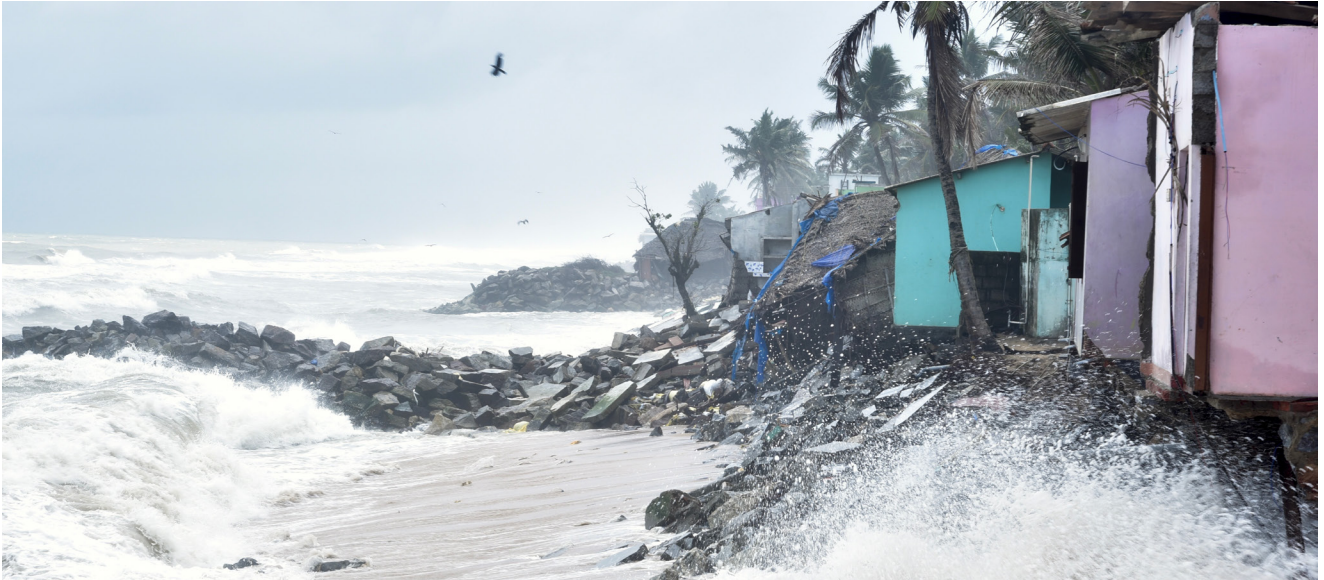
High swell waves hit the eroded shoreline of Anchuthengu, destroying houses, as a result of a storm in the Southern Ocean, 9000 km away from the Indian coast. (Photo: Kevin Julius)
