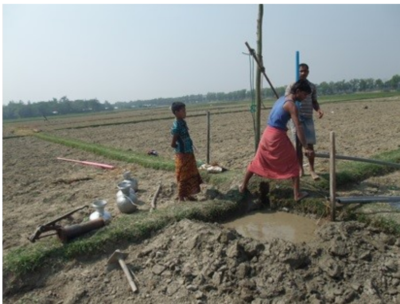
Figure 3: Installing a new hand pump
