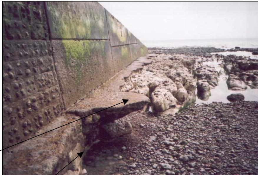
Part of the concrete plinth is left hanging in mid-air - level of platform would have originally been at this height.
