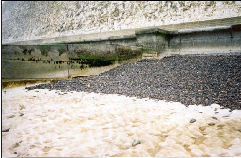
This continuous movement of shingle caused rapid downwearing and exposed a number of the MEM screws, which were then moved or bent. Site 20, the ridge MEM site located closest to the sea wall, was the first to be lost in November (figure 18), followed by 19 (also on a ridge) in March. Site 9 (20's runnel 'partner') may have been lost after November, but was never uncovered by the shingle again.
