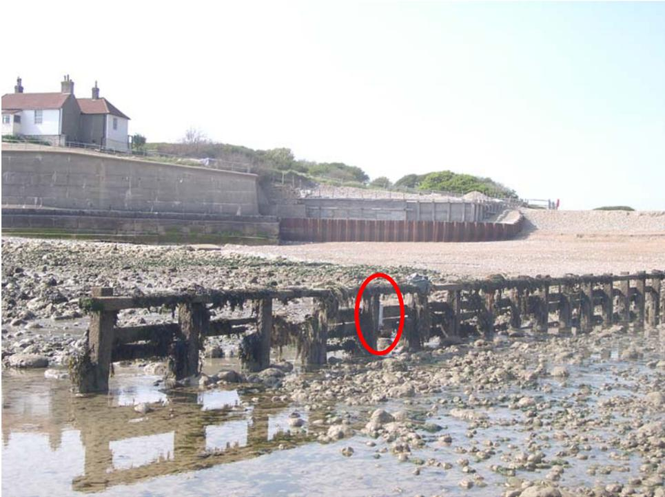
Figure 2: **Cuckmere Haven**. The recorder at Cuckmere Haven was installed upside down on the first suitable groyne pile at the end of the western groyne at Cuckmere Haven. The coordinates are  $x=551515.256$ ,  $y=97610.388$ ,  $z=-1.21$  m.
