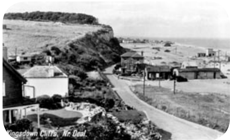
Postcard view of ca. 1950, showing greatly increased erosion.
