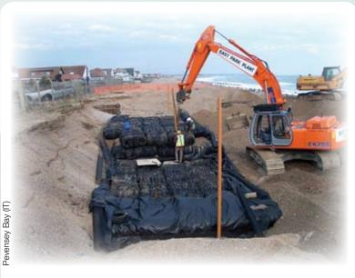
Novel ideas are being tried to strengthen our beaches and reduce the amount of shingle that needs to be brought in to recharge them. For example, bales of used tyres have been used to reinforce the beach at Pevensey.
