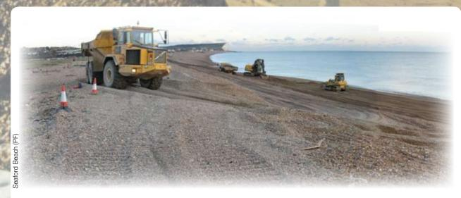
Once a beach has been 'recharged' with new shingle, the shingle will need to be 'recycled'. Lorries are used to move shingle back along the beach and the shape of the beach is rebuilt.
