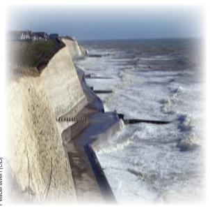
Breakwaters protect harbours, but can block longshore drift and have serious effects on beaches along the coast. The harbour at Dieppe traps shingle moving from the west, starving the beaches that protect houses to the east.
