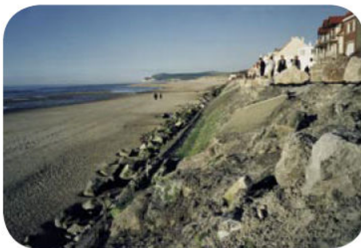
Very low beach levels in 2000. A concrete sea wall has since been built.
