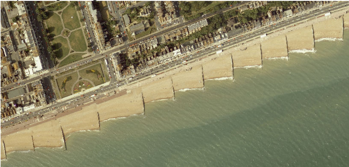
Groynes along Hastings beach
