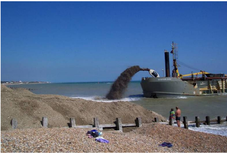
Beach recharge at Pevensey, East Sussex. Shingle is being pumped out from the boat onto the beach to build up its volume. The shingle was dredged from the bed of the Channel off Hastings.
